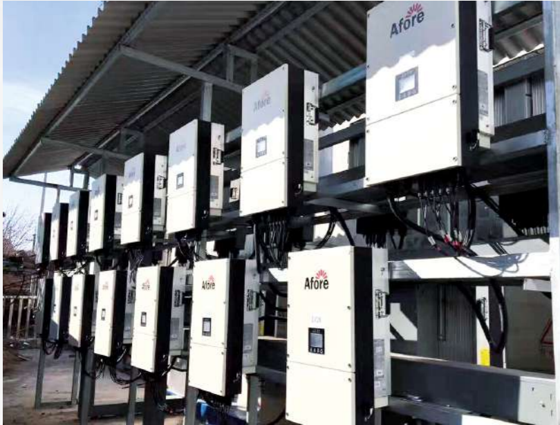
1.5MW Jiangsu, China
