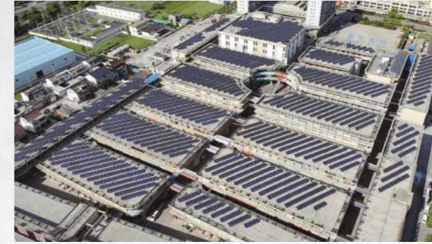
2.0MW Jiangsu, China
