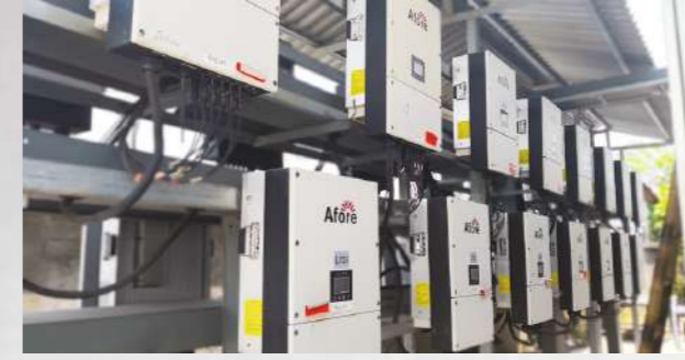
1.5MW Jiangsu, China
