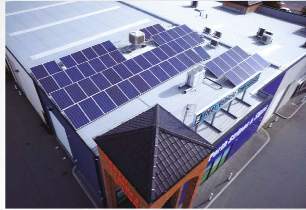
15kW Perth, Australia
