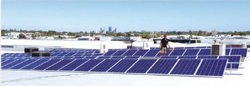
15kW Perth, Australia
